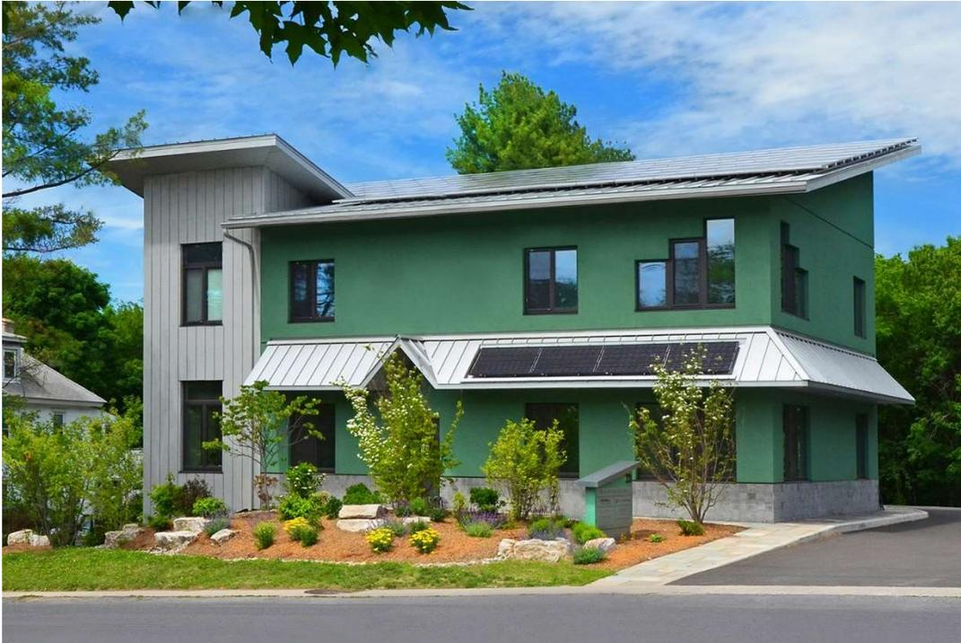
Front Façade of 231 Main St., New Paltz, NY, featuring 34.06kW grid-tied, roof mounted photovoltaic panels and transom windows
